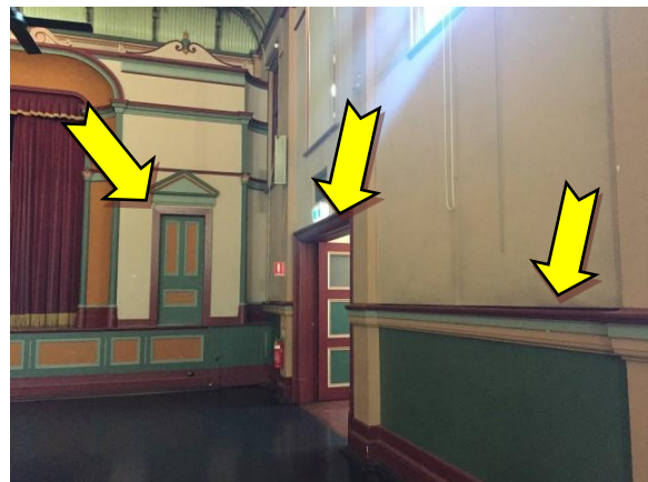
Photo 18. Interior, walls throughout – suspected lead-containing paint systems (red, dark green, peach, light peach, white, beige)
