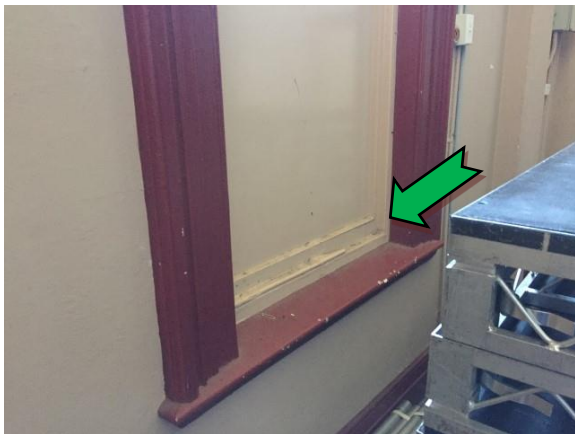
Photo 9. Ground level, main hall, east elevation, windows – non asbestos-containing window caulking
