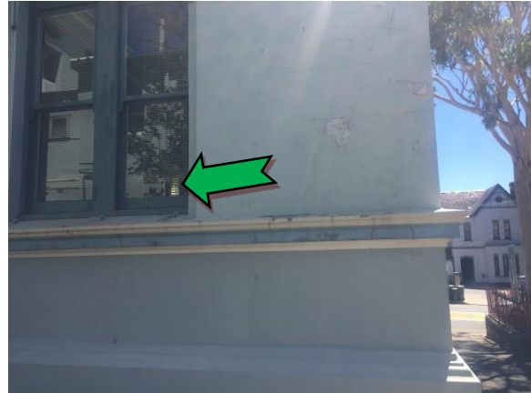
Photo 2. Exterior, throughout, windows – assumed non asbestos-containing window caulking
