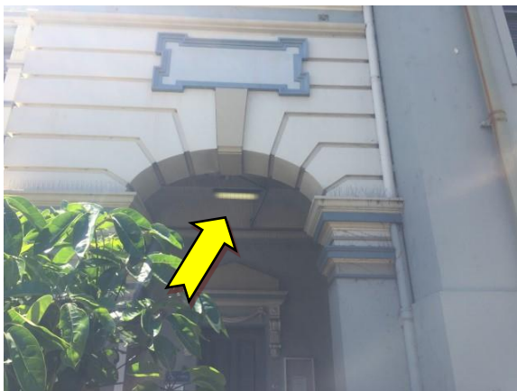
Photo 17. Exterior, southern elevation, disabled toilet – suspected PCB-containing single tube fluorescent light fitting
