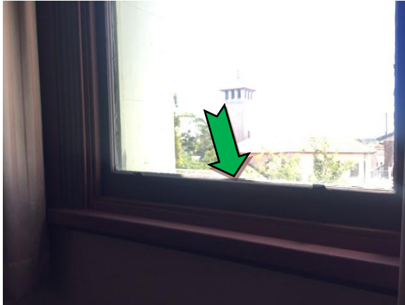
Photo 1. Exterior, level 1, reception room, windows – non asbestos-containing window caulking
